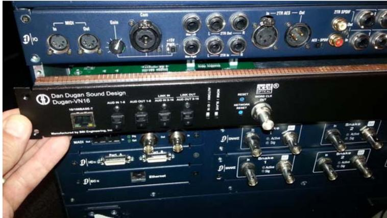
**Figure 2-22** Installing the Dugan-VN16 card in the FOH Rack
